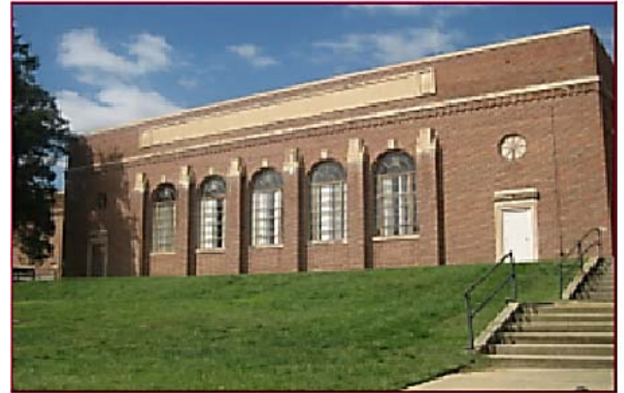
79-019-52 Old Marlboro Elementary School 14524 Elm Street
