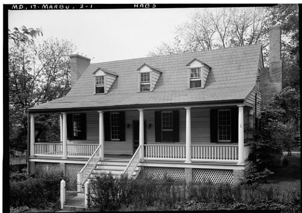
Wilson-Diggs House, Water Street Upper Marlboro – Moved to Lower Marlboro
