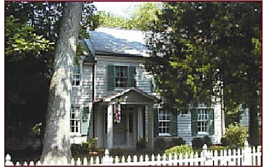
79-019-01 Thomas J. Turner House 14500 Elm Street
