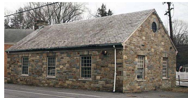
TELEPHONE SWITCH STATION
