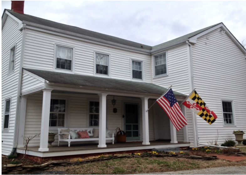
79-019-54 Bunnell-Anderson House 14509 Church Street
